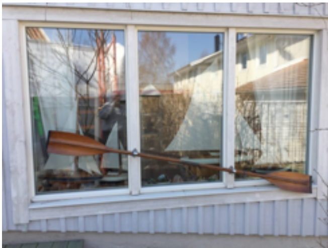
Window facing north
